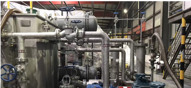
A Chemical Factory in Shandong, WSMH660-40, 10m 3 /h, 4.0Mpa, 40°C, transfer for coal tar
